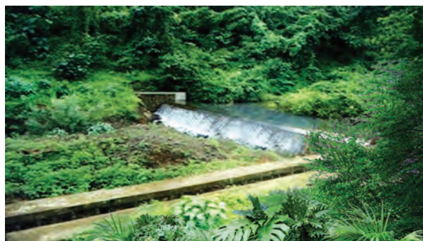
2.3.10 Diversion check dam
