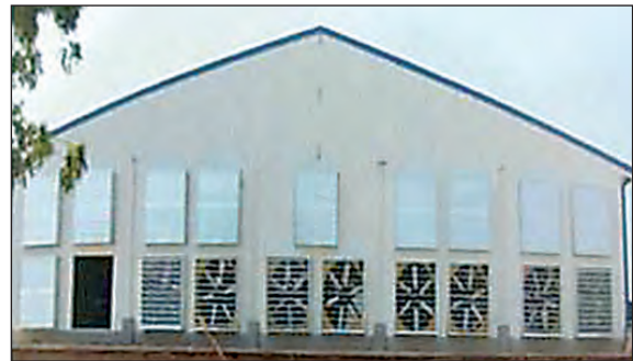
House with exhaust fans
