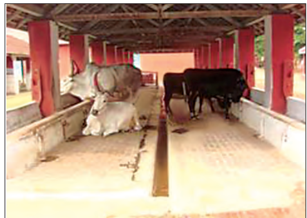
Fig. 2.12 : Brick floor of the conventional housing (Tail to Tail)
