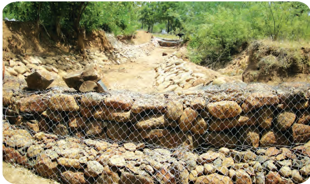
Fig. 6.12 : Gabion dam on stream
