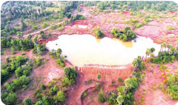
Fig.6.13 : Percolation tank
