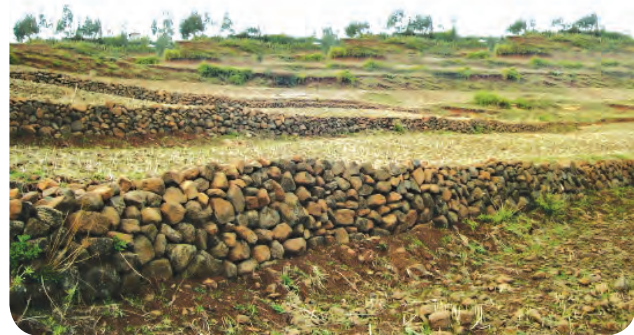
Fig. 6.10 : Stone contour bunding
