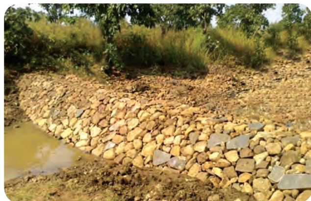
Fig. 6.11 : Loose rock check dam
