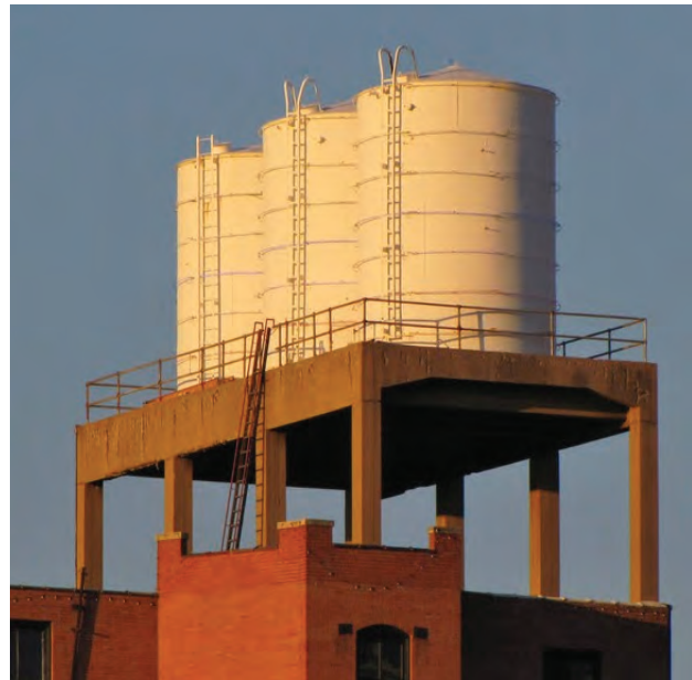
Overhead water tanks
